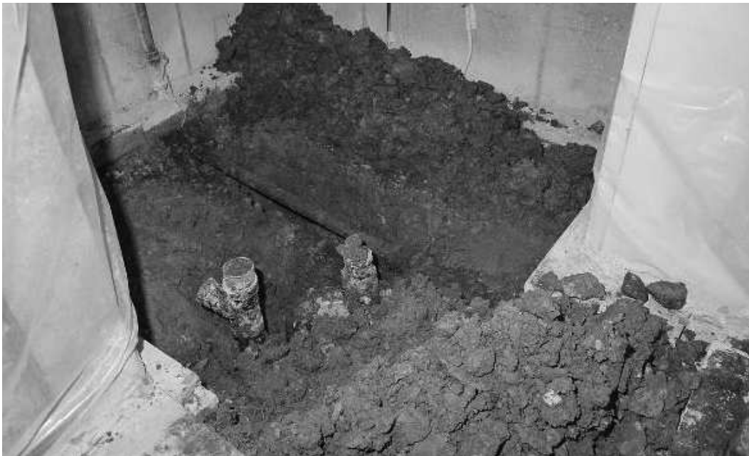
Figure 8. Photograph of complete excavation.
